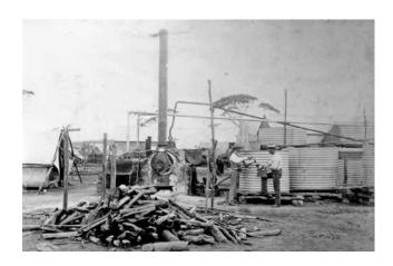
FIGURE 1 Western Australian Government water condenser, Coolgardie c. 1895, fuelled by timber supplied by cameltrains. The water was also distributed by cameleers (Image courtesy of State Library of Western Australia).
