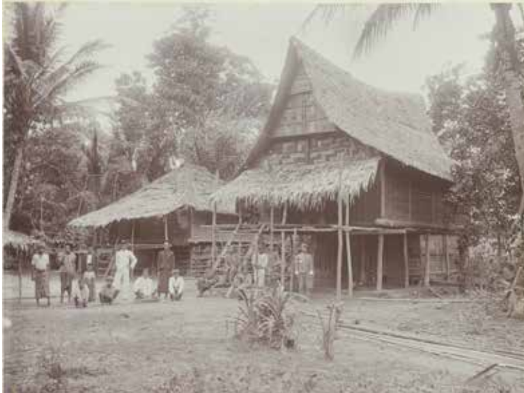
FIGURE 1 Indigenous Malay House in the Deli Region circa 1905. Photo courtesy of Leiden University Library, Leiden
