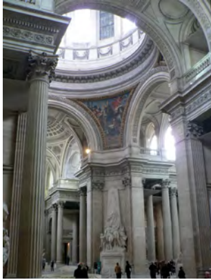
Fig. 4. The interior of the Panthéon showing the great piers supporting the dome, from which is suspended the pendulum. Photo by author.
