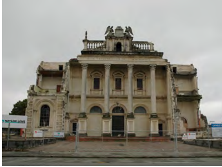
Fig. 2: Façade of the Cathedral of the Blessed Sacrament, Christchurch after further work to stabilize the structure after the collapse of the front towers. Photograph by Katrina Simon, December 2013.
