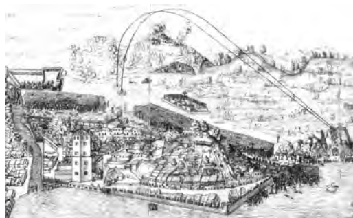
Fig. 2. Anonymous drawing dated 1568, showing Malacca under siege by the Acehnese. The city is defended by continuous stone ramparts punctuated by bastions affording the curtain walls flanking fire. By kind permission of Acervo da Fundação Biblioteca Nacional - Brasil. (Cart531967)
