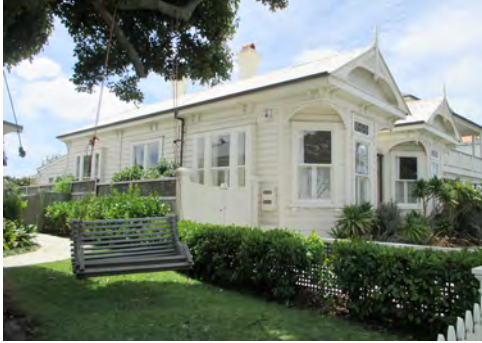
Fig. 3. Double bay villa at Devonport, constructed 1910. Used with permission.
