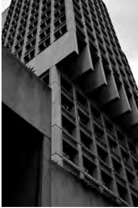
Fig 1. View from Kent Street.
