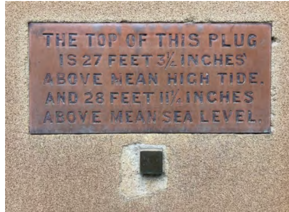
Figure 2. Datum plug and plaque embedded in the Bridge Street façade. Photograph by the author.
