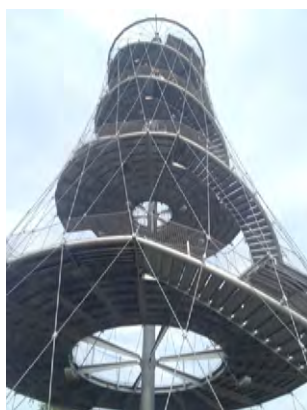
Fig. 3. Killesberg tower designed by Jörg Schlaich, Stuttgart, Germany (2000).
