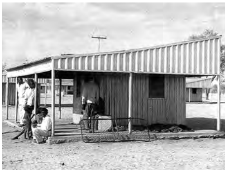
Fig. 4. Lysaght Kingstrand Transitional House Stage 1 at Amoonguna, N.T., 1965, (Photograph by Balwant Saini in "Aboriginal Housing State of the Art, non-State of the Art," Architecture Australia, 77 [1988] 36.
