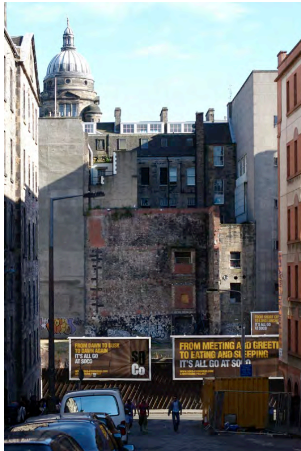
Figure 4. View of vacant SoCo site from the Cowgate level, with the Category A-listed dome of the University of Edinburgh's Old College in the background. Source: Tom Parnell, Flickr, 2009.
