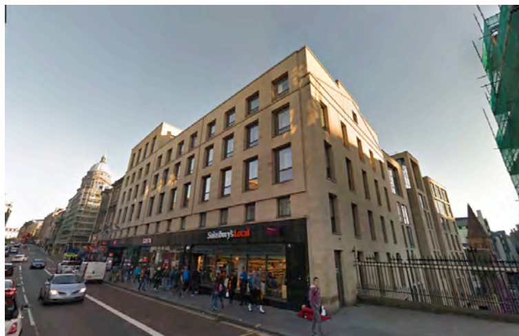
Figure 6. South Bridge elevation of completed SoCo development, with the bridge over the Cowgate and Cowgate façade shown in right of image. The Category A-listed Old College dome is visible in the background. Source: Google Street View, 2017.
