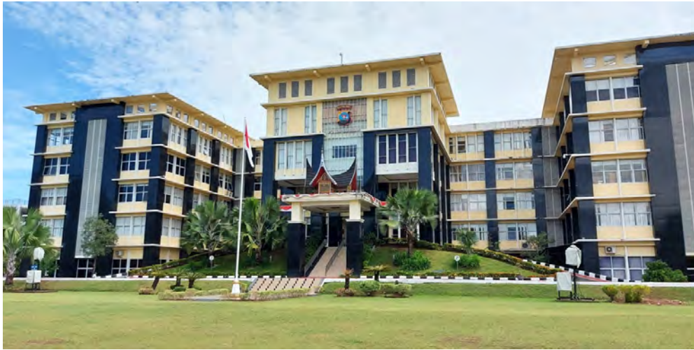
Figure 3. The new Regional Police Headquarters of West Sumatra. Bagonjong roof was added to the drop-off roof as requested by the governor (Photograph by Rr. Diah Asih Purwaningrum, 2022).
