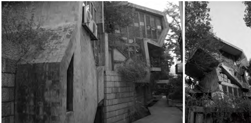
Figure 8. The Taihu rock houses in the Southern Song Imperial Street renovation project, Hangzhou, 2007-09 (Photograph by Xin Jin).
