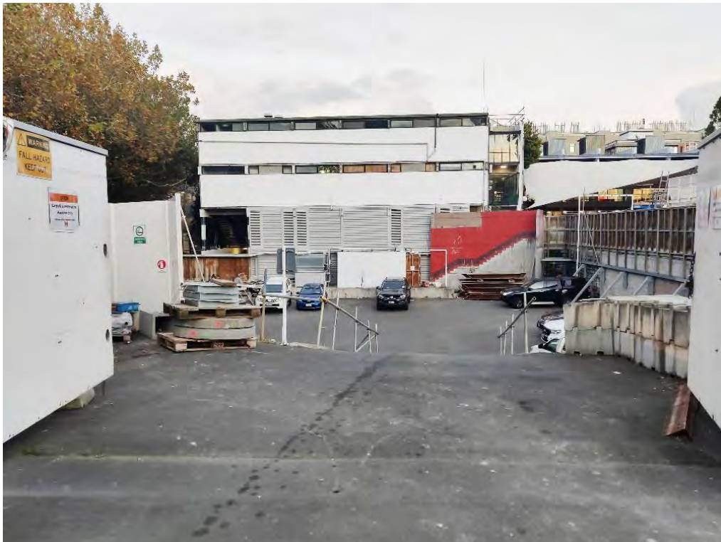
Figure 6. Maidment Theatre demolition plot, 2022 (Candida Rolla).
