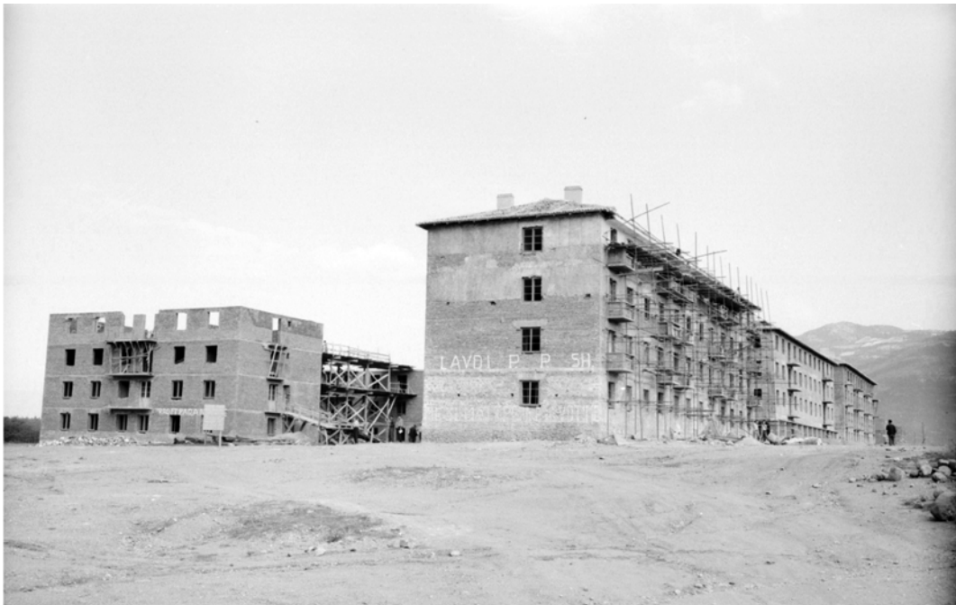
Figure 2. The first housing block (lagje nr. 1) under construction in the new town of Kukës. The graffitied words “Lavdi P.P.SH.” on the wall means “Glory to the Albanian Labour Party”; P.P.SH is the acronym of “Partia e Punës e Shqipërisë” (Courtesy of Arkivi Qendror Teknik i Ndertimit, AQTN, Fototeka, v. 1964).
