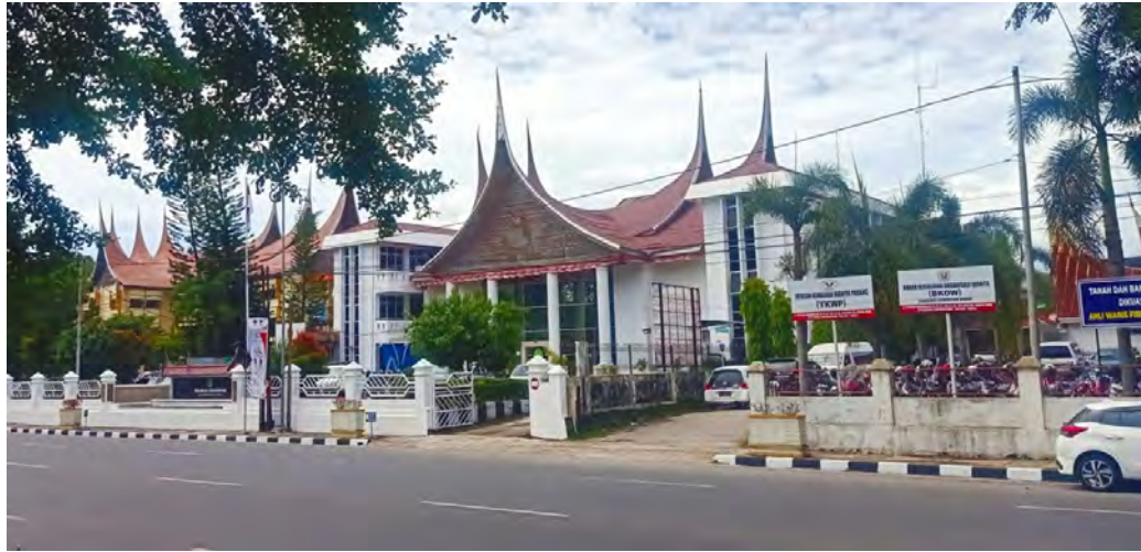
Figure 2. The pointy skyline on one side of Jalan Sudirman street, Padang, as the governmental street corridor (Photograph by Rr. Diah Asih Purwaningrum, 2022).
