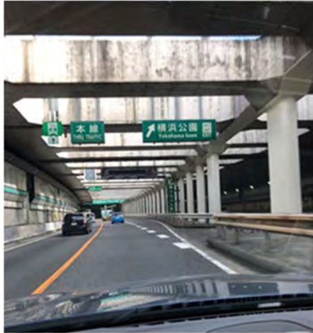
Figure 17. Completed open-cut motorway near Yoshida canal in 2019 (Photograph by Toshio Taguchi).
