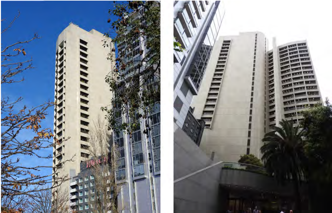
Figure 5. Shell House, Melbourne (1985-88), views from Spring Street and Flinders Lane. Architect: Harry Seidler and Associates (Photographs by Giorgio Marfella).
