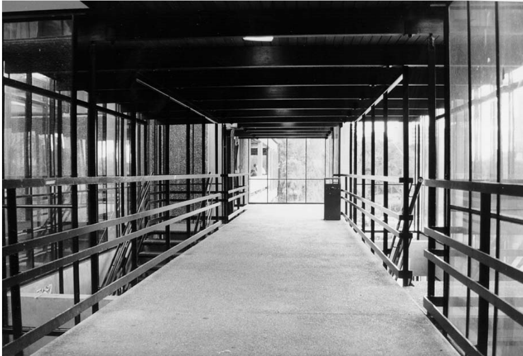
Figure 4. Student Union Building, 1999 (Salmond Architects).
