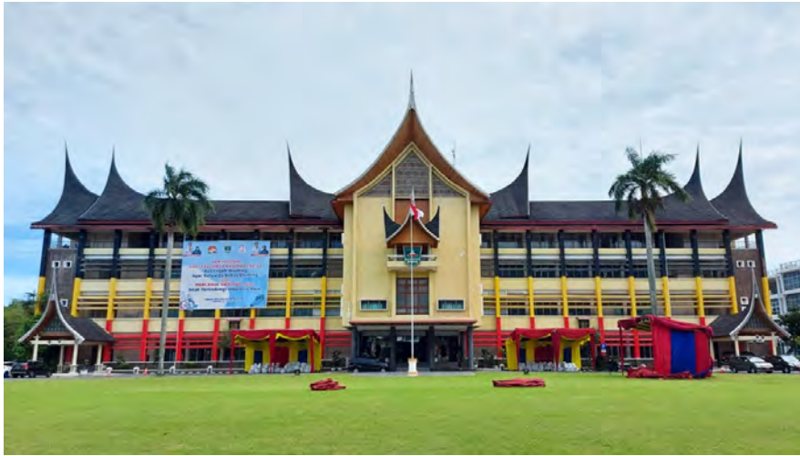
Figure 1. The West Sumatra Governor Office, or Rumah Bagonjong, was the first modern building that adopted a Bagonjong roof in the region (Photograph by Rr. Diah Asih Purwaningrum, 2022).
