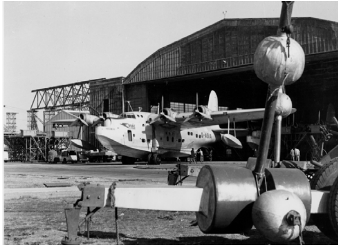
Figure 4. Image of the enormous industrial hangars that took over a large portion of Lyne Park. The hangars were large enough to house flying boats while they were under repair (“Rose Bay 1940s,” Qantas Heritage Collection).
