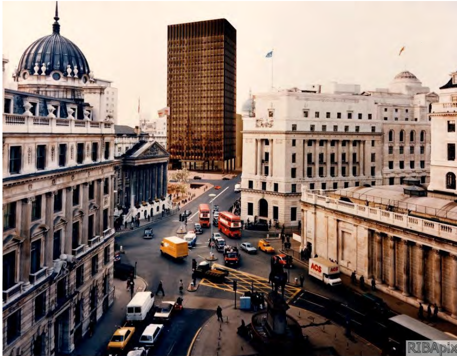
Figure 2. Mies van der Rohe's Mansion House Square tower proposal (RIBA 28878, John Donat / RIBA Collections).
