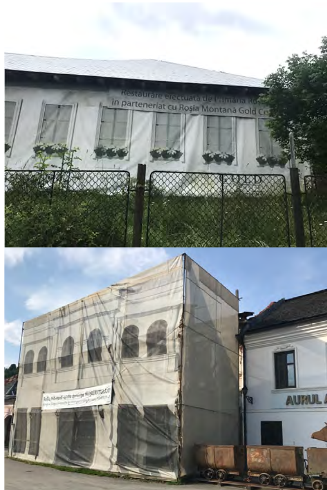
Figure 4. Top image: The message reads: “Rehabilitation by Roșia Montană Town Hall partnered with Roșia Montană Gold Corporation” (tense of the message suggests the rehabilitation has been completed, however in 2017 there was still a canvas to the main façade). Bottom image: “Rosia Montana exists because of MINING! Help us keep a valuable tradition of Apuseni mountains, MINING!” (Photographs by Alexandra Florea).
