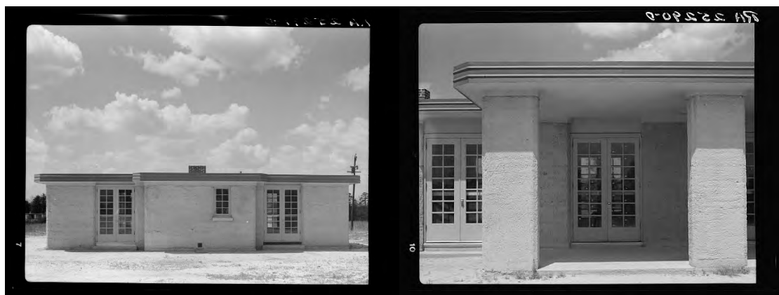
Figure 1. Hibben's rammed earth houses at Gardendale Grand Olive, Alabama. Source: Library of Congress, Prints & Photographs Division, FSA/OWI Collection. Reproduction number: (right) LC-USF34- 025290-D [P&P] LOT 1611, (left) LC-USF34- 025291-D [P&P] LOT 1611.
