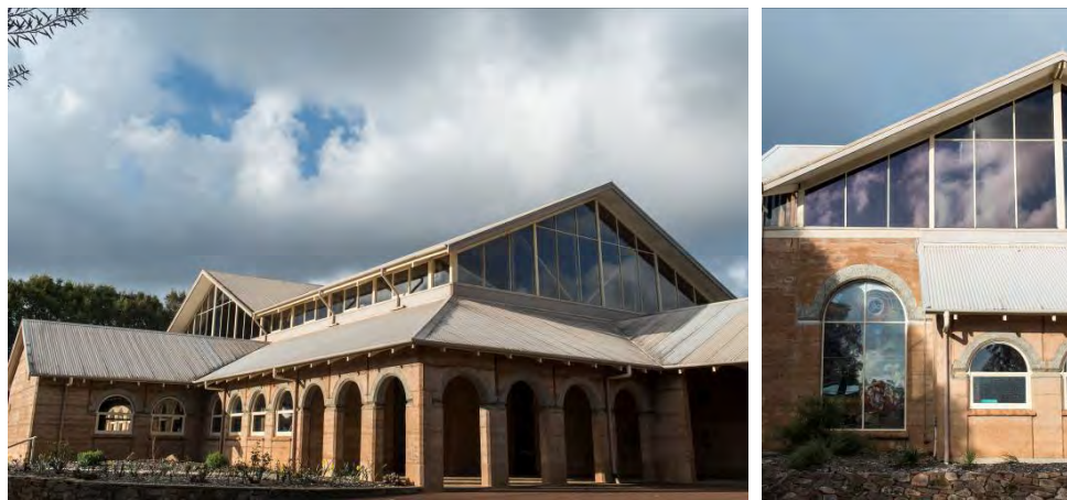
Figure 5. Saint Thomas More Catholic Church. Built in 1983, Margaret River. Photographs V. Strazzeri.
