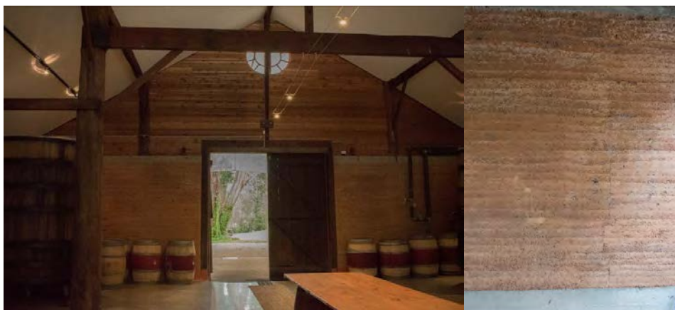
Figure 2. (L) original building at Cape Mentelle built 1977; (R) detail of the wall. Photographs V. Strazzeri.
