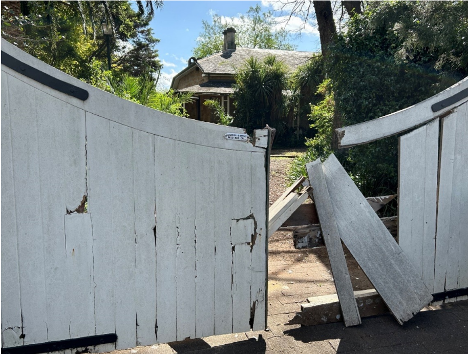
Figure 1: Wavertree, Parramatta, New South Wales, designed by James Houison (1800–1876). (Photograph by Paul Hogben, September 2024)
