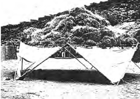
Fig. 6. Architectural experiments included the use of local materials such as spinifex grass. Aboriginal Environments Research Centre.
