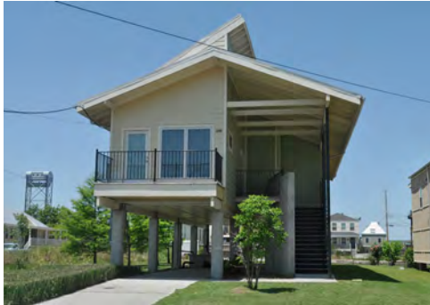
Fig. 6. an example of the Constructs' design with recessed front entry and interior-accessible front porch (Photograph by author.)
