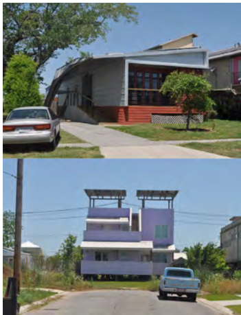
Fig. 3. MIR houses differ greatly from the historic fabric of the city, not just in appearance, but in scale and the way in which they address the street – two important factors in retaining a sense of neighbourhood which existed pre-Katrina. Photographs by Michael Kahn.
