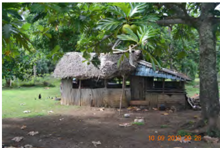
Fig. 10. Elevation of Kaho's Tongan kitchen now clad in corrugated metal, author September 2013.
