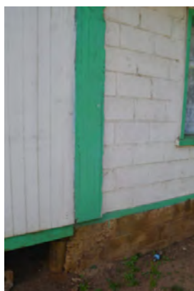
Fig. 4. Junction between Sioeli's cyclone house's timber stumps and concrete block addition's perimeter wall, author September 2013
