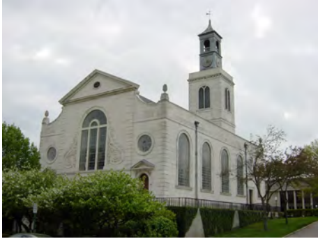
Fig. 2. Christopher Wren and Robert Hooke, St. Mary Aldermanbury, east end, built in London, England, 1671–81, destroyed during bombing raid, 1941, ruins moved and rebuilt at Westminster College, Fulton, Missouri, USA, 1965–69. Photograph by Keith Eggener, 2013.
