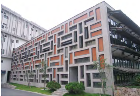
Fig. 2: Fig. 2 Teaching Building no. 21 in Phase II, Xiangshan Campus (2007). Photograph by Hing-wah Chau.
