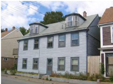
Fig. 2: The 'Scottish' or five-sided dormer can be seen here in a timber-framed and clad house on Church Street in Pictou. Photograph by Amy Clarke, 2012.
