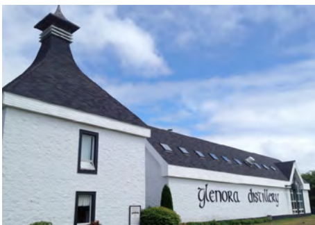
Fig. 5: The white-washed walls and pagoda roof of the Distillery are visible from the visitor car-park. Photograph by Amy Clarke, 2012.
