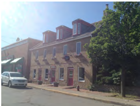
Fig. 1: The 'Scottish dormer' or five-sided dormer element, seen here at 110 Water Street, Pictou, is one of the most commonly mentioned 'Scottish' architectural features of Nova Scotia. The combination of the five-sided dormer with a neoclassical stone dwelling such as the one pictured is quite unusual in Nova Scotia, and outside of the town of Pictou the dormer is typically found in timber structures. Photograph by Amy Clarke, 2012.
