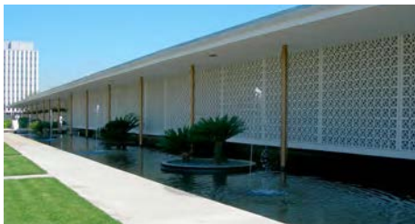
Fig. 1. Stuart Pharmaceutical Co., Pasadena, Calif., by Edward Durrell Stone, 1956. Photograph by Robert Skolmen. Wikimedia Commons.
